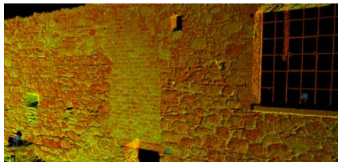
Point Cloud Image – Wall Detail
