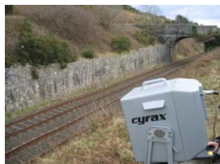
Wellington Cut retaining wall
